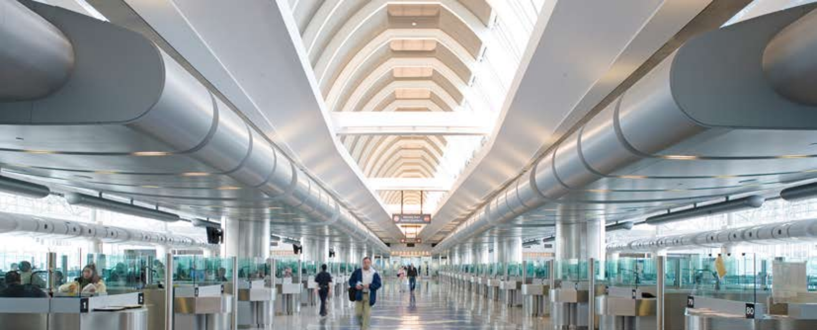
Air Cooled Screw Chiller
